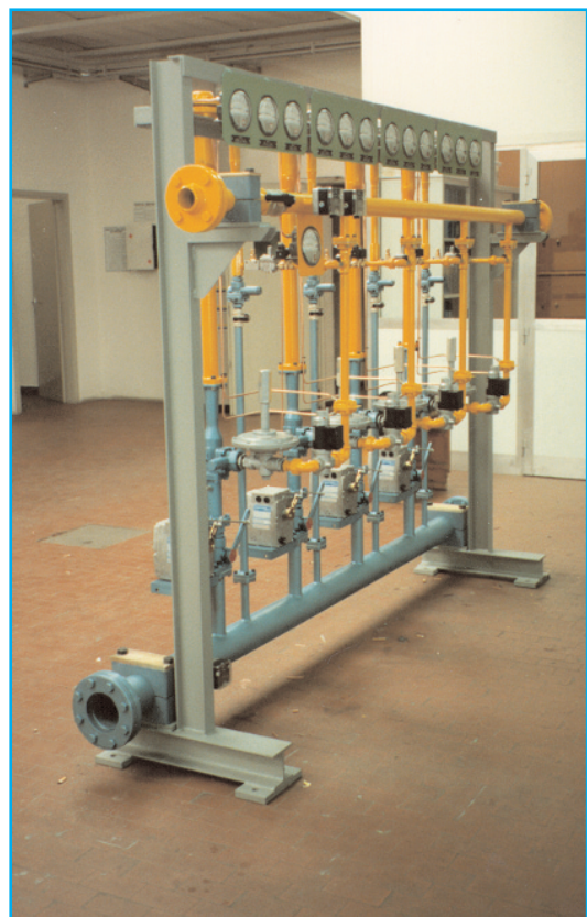
Pre-assembled group for pressure adjustment and control for pre-mix burners (Barilla)
