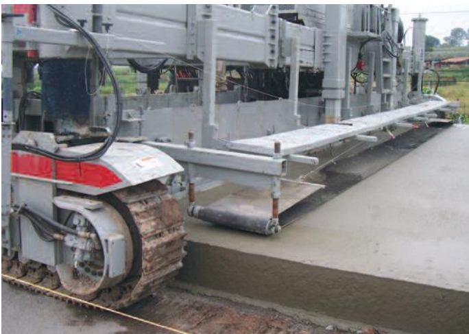
Optional belt finisher enhances the pavement surface.
