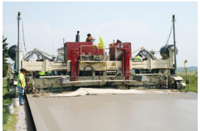
3-D Controls allow the SF-3000 to pave without stringline. This provides better access for the concrete trucks, other equipment, and the finishing crew.
