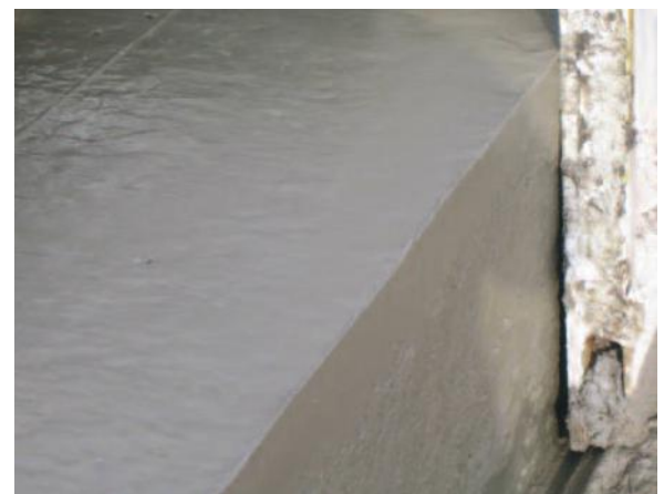
Everything works together to create pavement with smooth flat finish and a sharp square edge.
