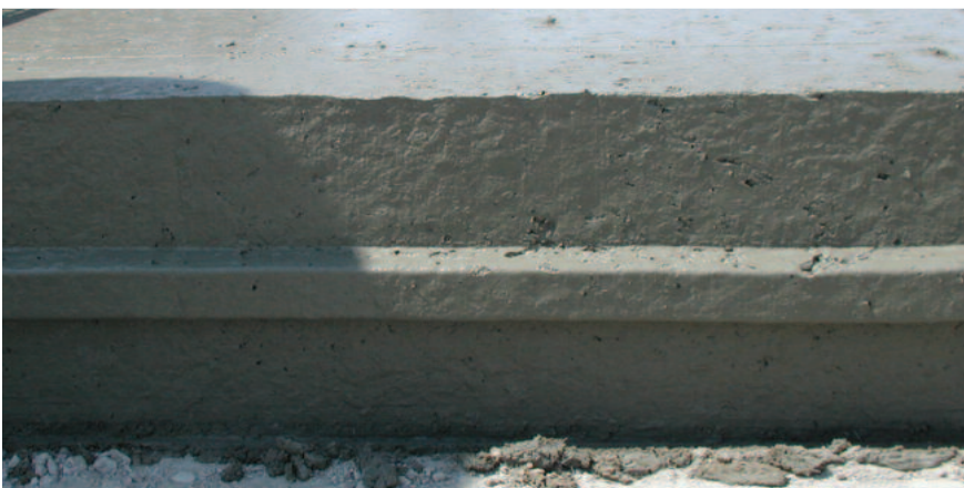
Edge of pavement with optional key-way inserter (top), and optional male key-way block-out (bottom).
