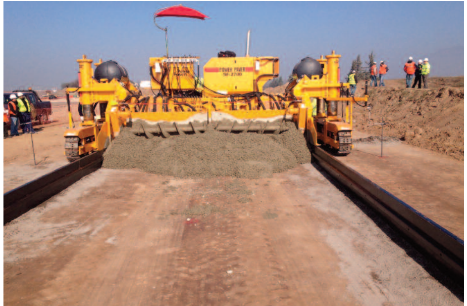
The SF-2700 frame can be extended to pour over fixed forms.
