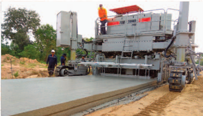
▲ Power Curbers 7700 Multipurpose Slip-Form Machine Paving
