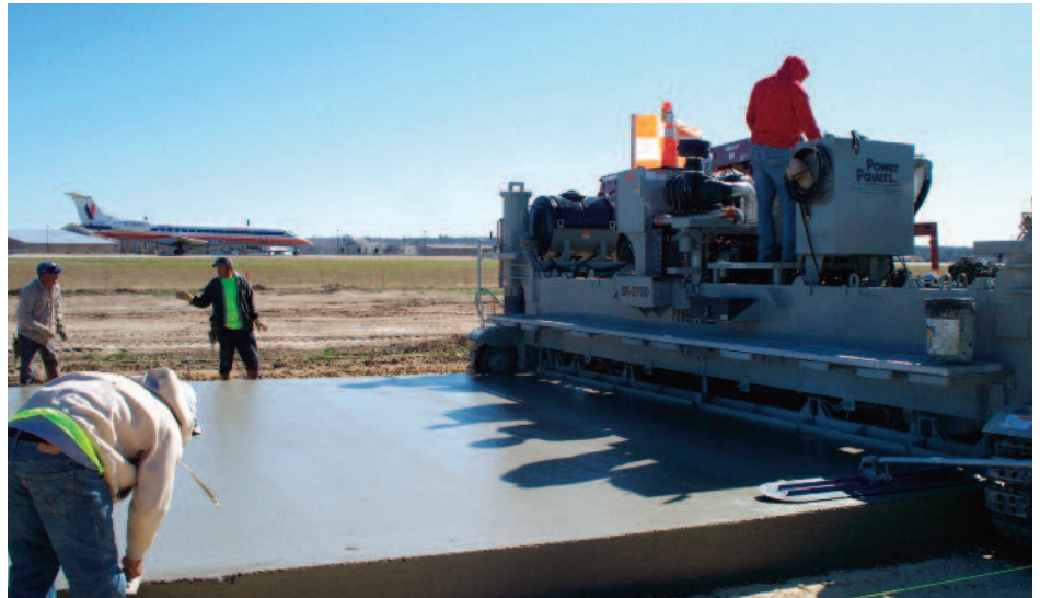
SF-2700 paving an airport.
