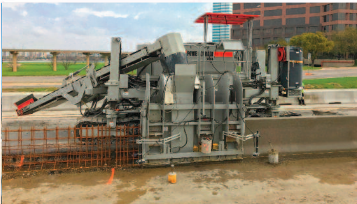
▲ Power Curbers 7700 Multipurpose Slip-Form Machine Pouring Barrier
