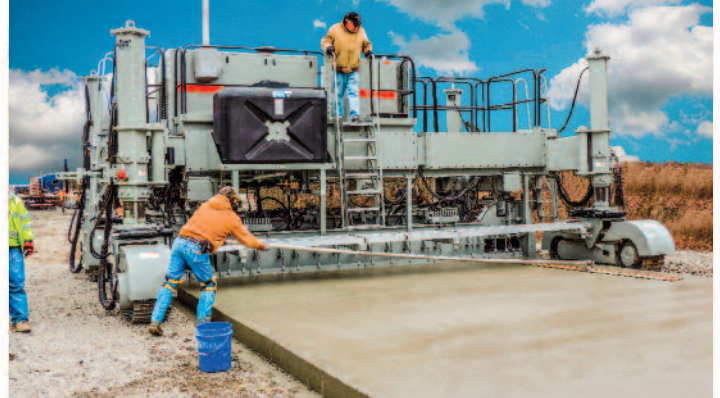
▲ Power Pavers Full-Sized, 4-Track SF-2404 Slip-Form Paver
