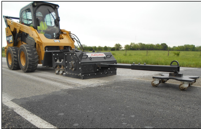
Corrective Grind—IRI Improvement
