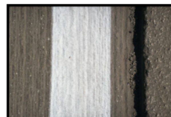
Micro Milled Surface-Ready for Traffic
