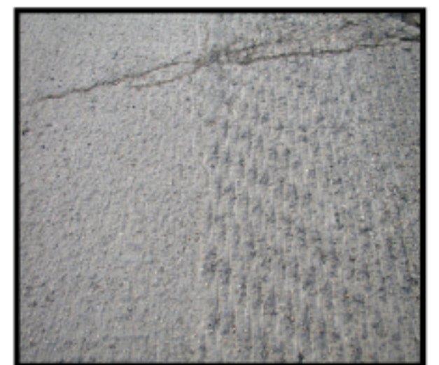
Micro Milled Surface Fine Milled Surface
