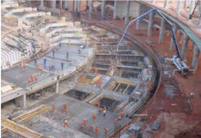
Construction of intermediate and perimeter drop beams
