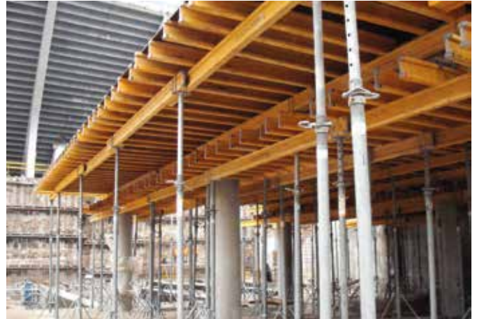
Wooden beams at different levels
