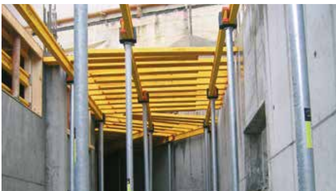
Formwork against a single wall
