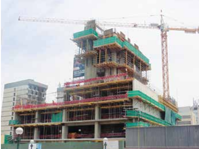
Shoring with certified EP steel prop
