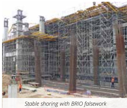
Shoring on a building construction with G falsework
