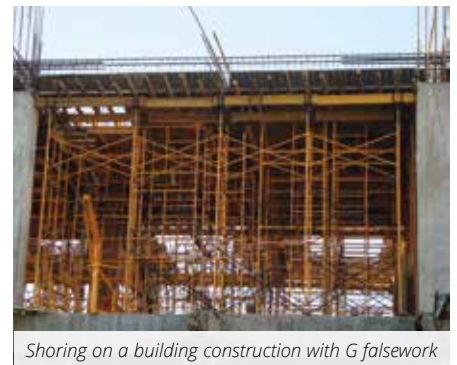
Formwork assembly platforms on falsework tower
