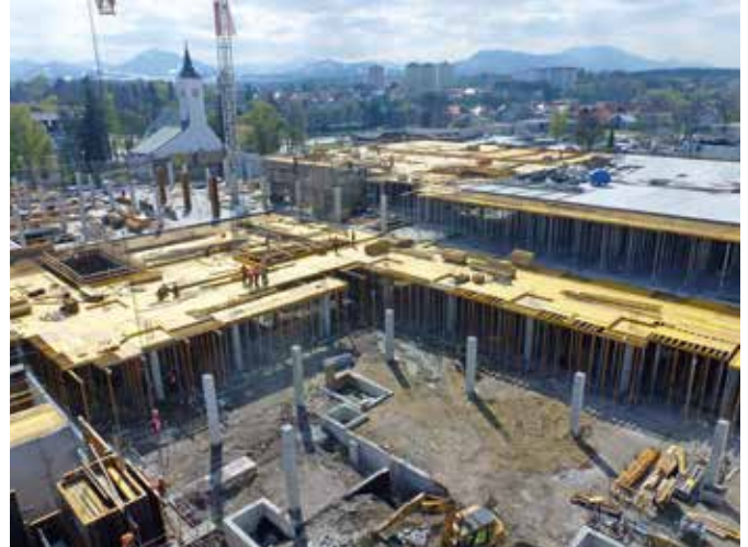
Shoring with SP prop
