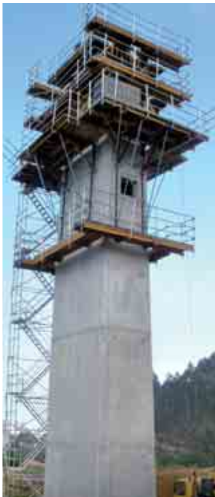
CR-250 brackets in pier execution with pouring, intermediate, main and cones recovery platforms. The access is provided by BRIO scaffolding ladder
