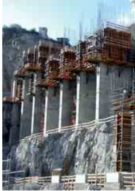
Climbing bracket used in building and civil engineering
