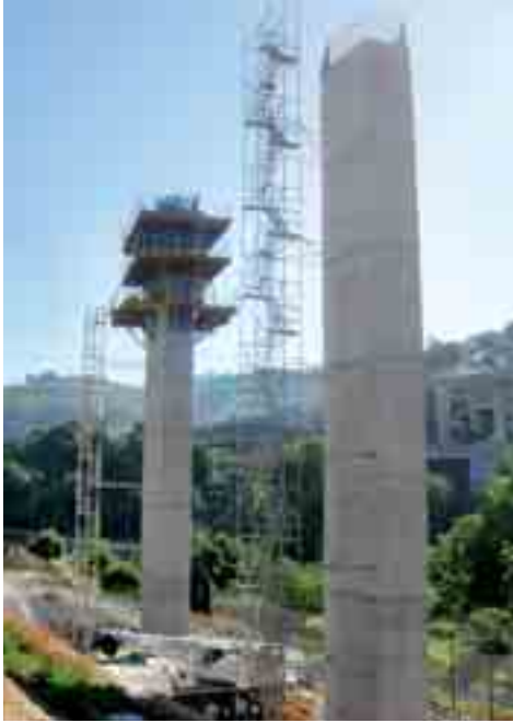
Climbing bracket used in building and civil engineering
