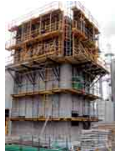
CM-220 brackets with ORMA vertical formwork
