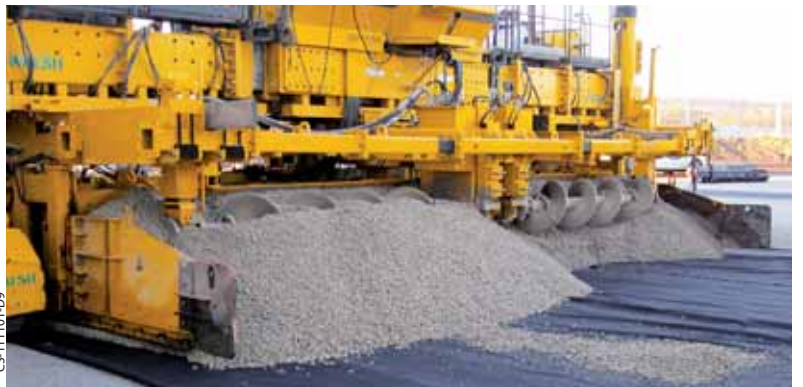
The PS-2600 is placing and spreading cement treated base. Its 7500 series placer mold has 10 inches (3.05 mm) of vertical adjustment with hydraulic cylinders.
