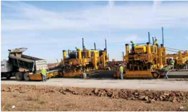
The GOMACO paving train consists of the PS-2600 and GHP-2800 using the Topcon 3D machine guidance system.
