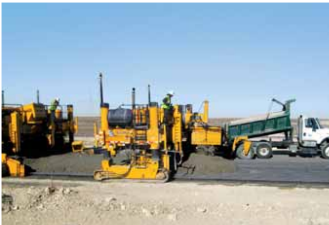
The GOMACO PS-2600 has a belt conveyor length of 22 feet (6.71 m) with a width of five feet (1.52 m).
