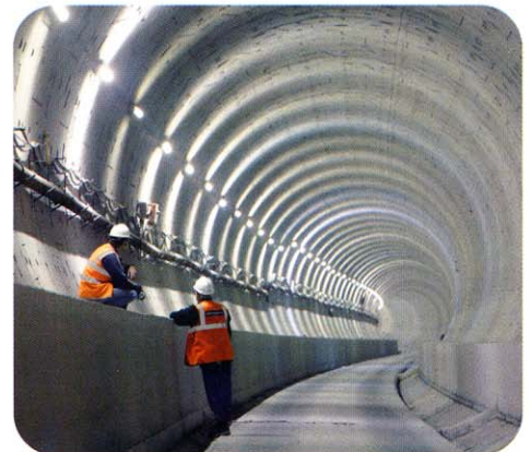
The profile of the track bed floor and walkways shows how challenging it was to slipform the three different profiles.
