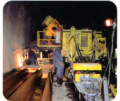
Anti-Derailment Upstand on Taiwan's high-speed rail.
