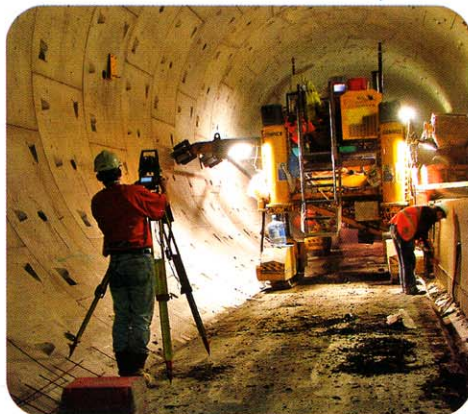
The profile of the track bed floor and walkways shows how challenging it was to slipform the three different profiles.
