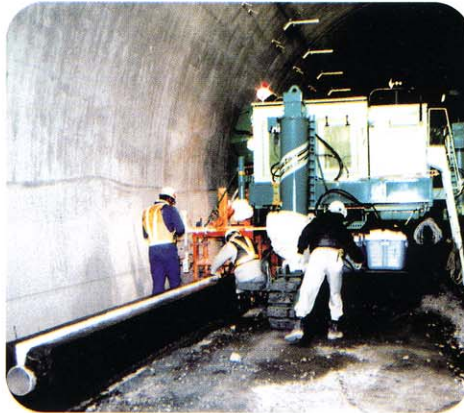
Anti-Derailment Upstand on Taiwan's high-speed rail.
