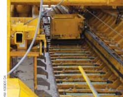
**1:** The bar loading trolley places a bar into each individual bar loading tray across the entire width of the new pavement.
