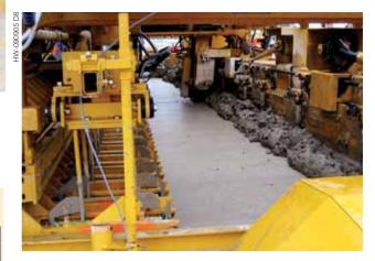
**5:** The IDBI attachment's finishing process includes a tamper bar, unique oscillating straightedge, paving pan and stainless that follow the bar inserters and repair the scarring from the insertion process.
