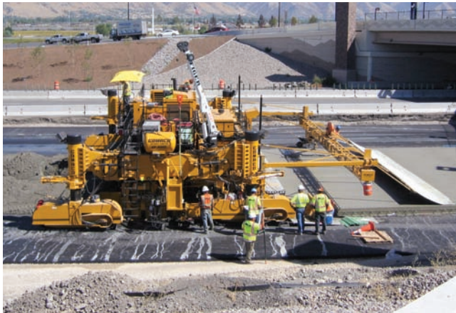
The GOMACO GP-4000 with independent IDBI attachment slipforms 36 feet (11 m) wide on an interstate project.
