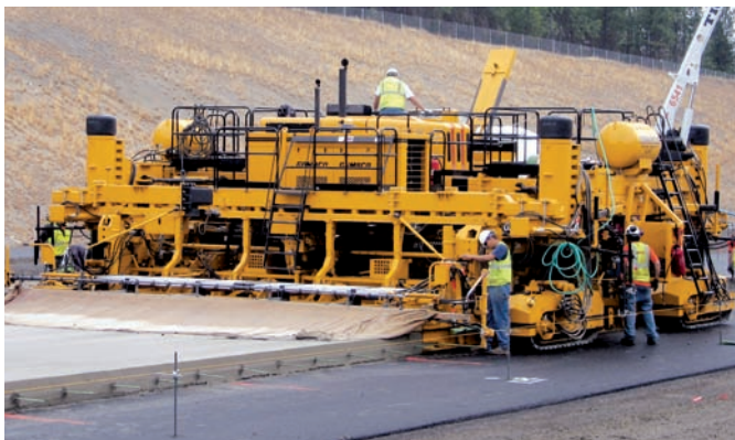
The IDBI attachment is capable of widths as narrow as 10 feet (3 m) and as wide as 50 feet (15.2 m).
