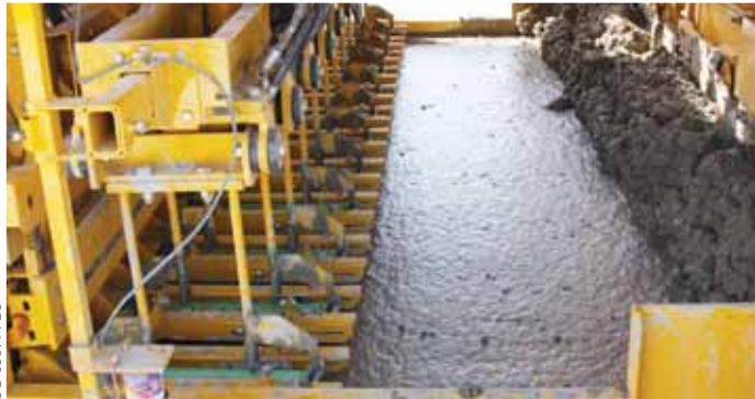
Patented insertion forks provide the industry standard in bar placement accuracy.
