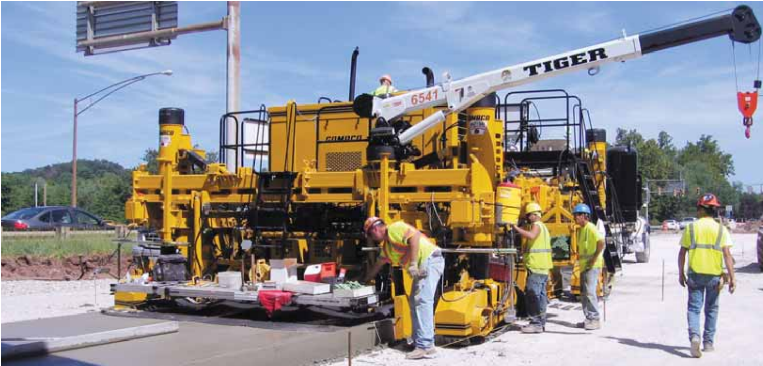
The Commander III features the 3100 series open-front mold with auger and adjustable stainless providing the superior GOMACO finish.
