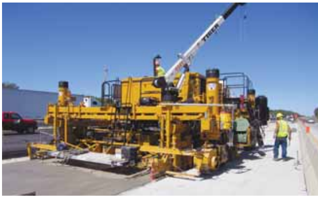
A scab-on, single lane rehabilitation project.
