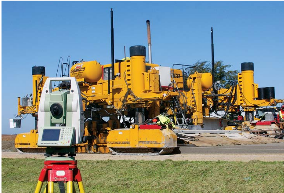
The project was slipformed half-width and one lane of traffic was kept open at all times using flaggers and pilot cars to direct the vehicles.
