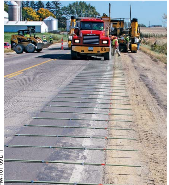
#5 steel rebar, six feet (1.8 m) long, were placed on 30 inch (762 mm) centers on the existing roadway to tie on the new eight inch (203 mm) thick shoulder.
