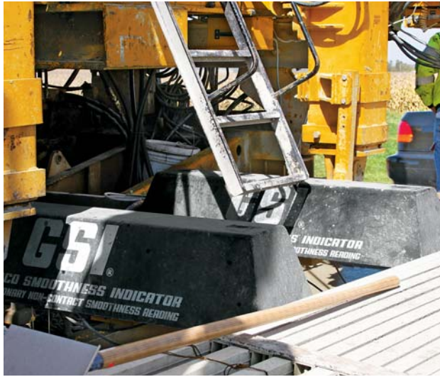
Paver-mounted GSI units provide instant rideability results. The GSI is GOMACO's proprietary non-contact profiler capable of providing instant smoothness results.
