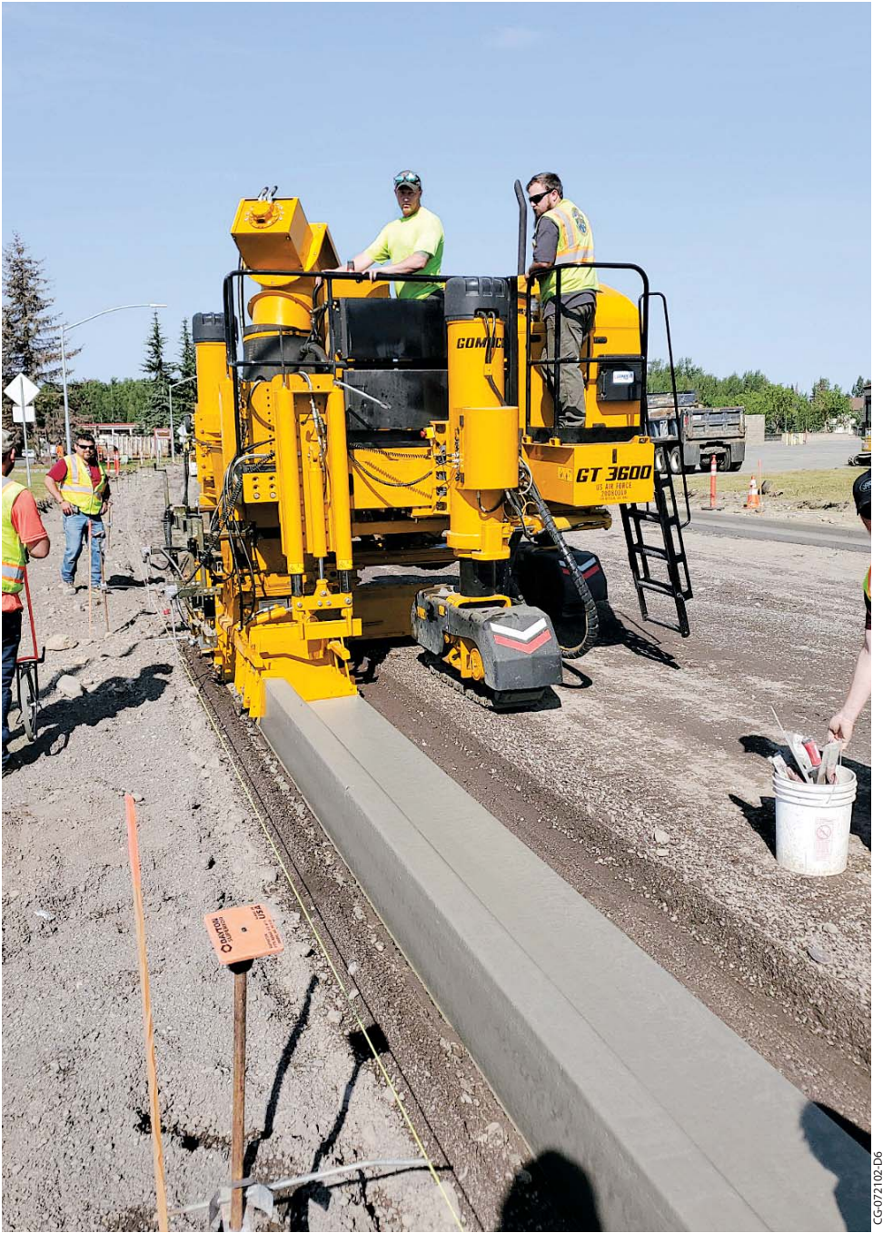
The exclusive, independent adjustable stainless steel troweling section seals and provides the superior GOMACO finish.
