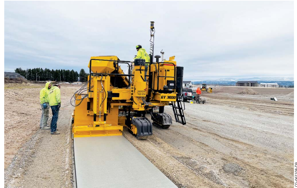
The operator's platform and safety railing telescope out with the sidemounted mold to give the operator visibility over the entire operation. This GT-3600 is slipforming a five foot (1.52 m) wide sidewalk.
