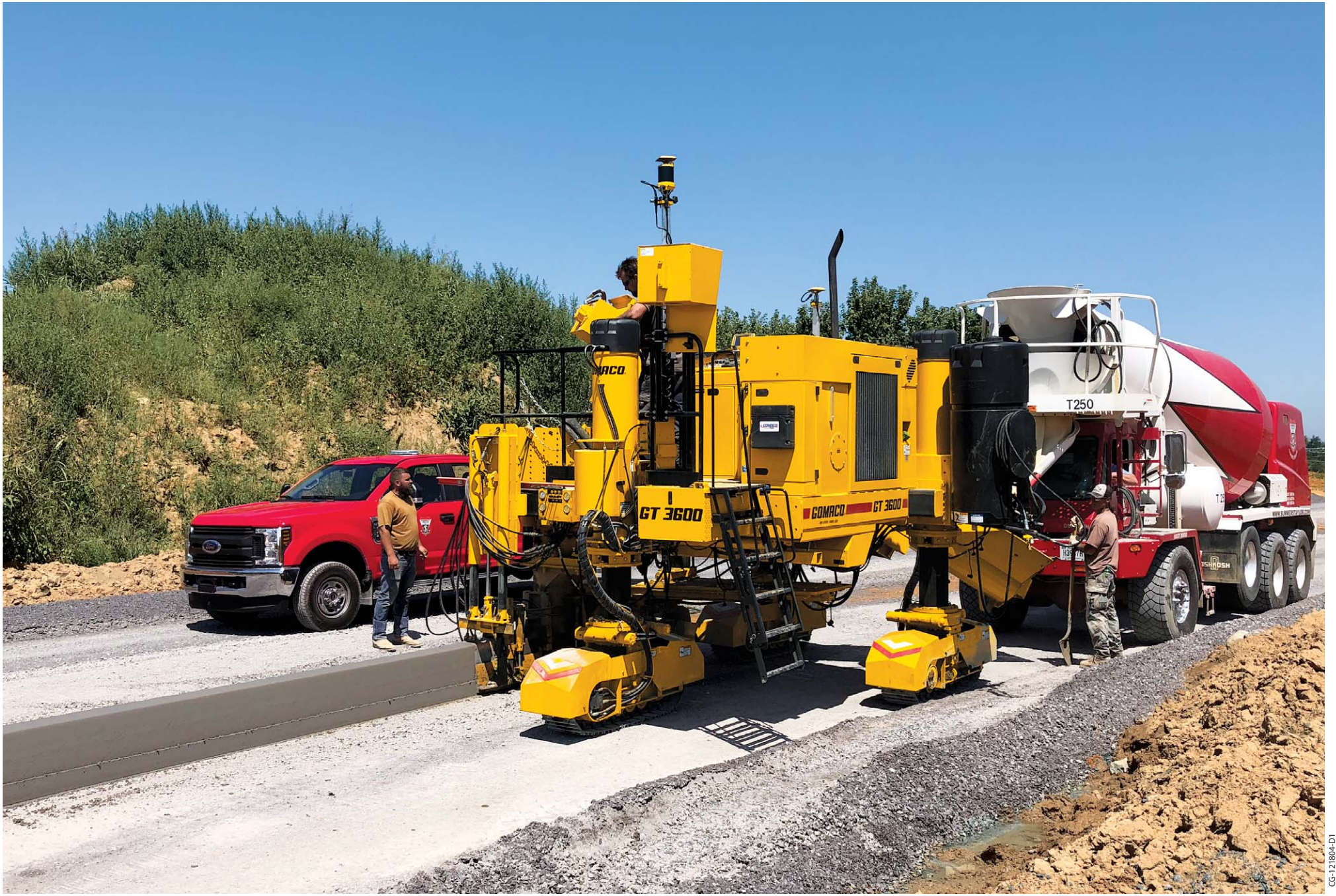
The GOMACO Xtreme GT-3600 is slipforming an 18 inch (457 mm) stand-up curb and is equipped with the GOMACO Remote Diagnostics (GRD) allowing for remote upgrades and fleet management from a cell phone or laptop computer.
