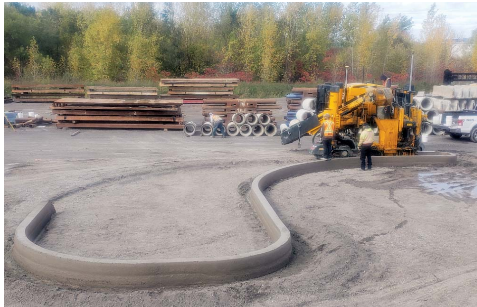
The Xtreme GT-3600 slipforms a stand-up curb with tight radii using 3D machine guidance.
