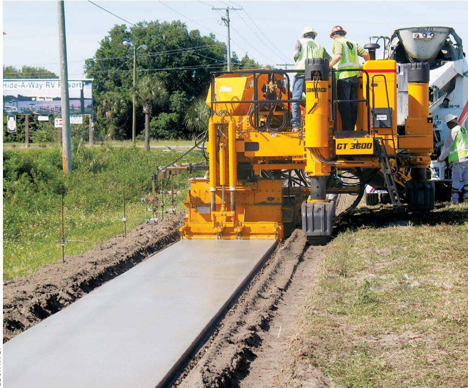
All-Track Positioning (ATP) provides easy setup for slipforming sidewalks. This GT-3600 is slipforming a five foot (1.52 m) wide sidewalk with a side-mounted mold.
