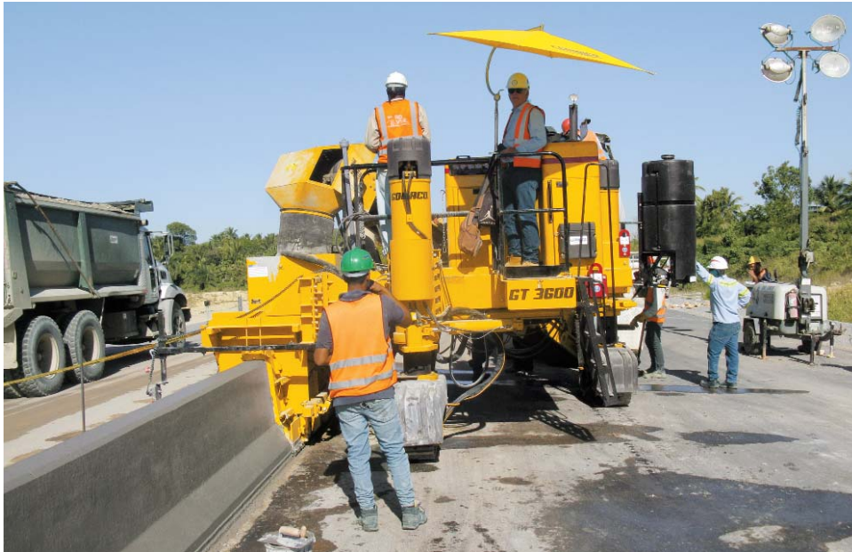
The optional sidemounted barrier and parapet attachment allows the GT-3600 to pave a maximum height of 50 inches (1270 mm).
