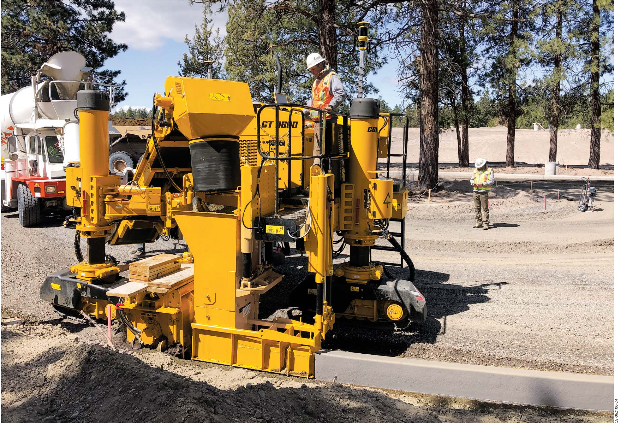
Repeatable mold offset is accomplished through G+ and a smart hydraulic cylinder for telescoping the mold mounting system.
