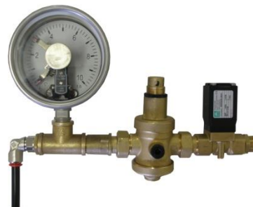
Control armature of the seal cooling medium
