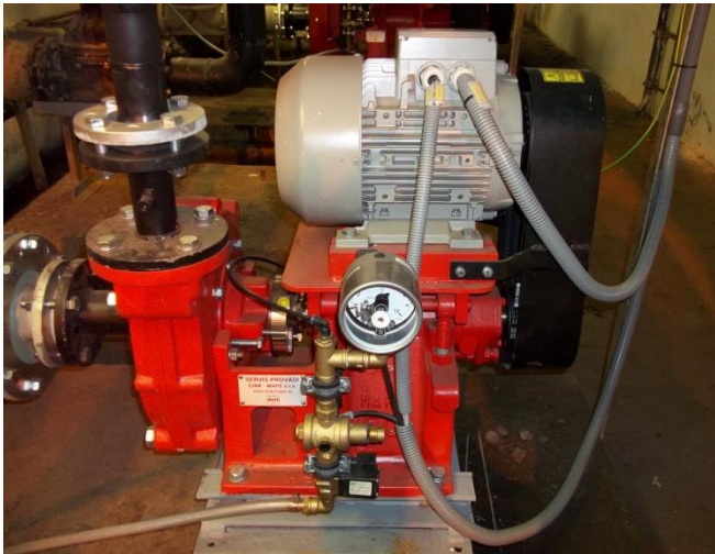
MAPE 50, Water treatment plant – transportation of water with sludge. Installation of the Automatic seal protection ASP 21
