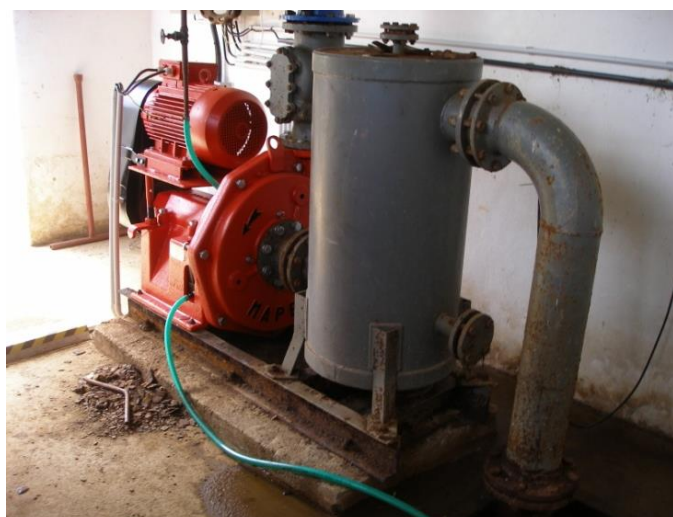
MAPE 100 Transportation of sludge water. Installation of countershaft tank
