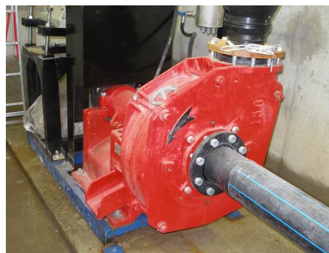
MAPE 150, Transportation of sludge water
