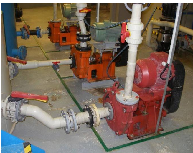
MAPE 50, Transportation of aluminium sulphate during the manufacturing process
