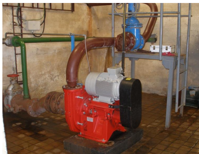
MAPE 100, Transportation of sediments from sand traps
