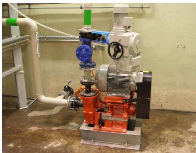
MAPE 50, Dredging station - mixtures of water with slag
