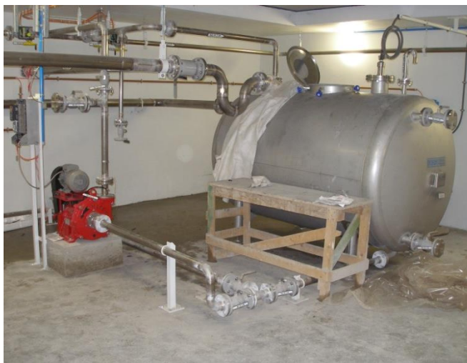
MAPE 50, Nuclear power plant. Transportation of liquid radioactive waste
