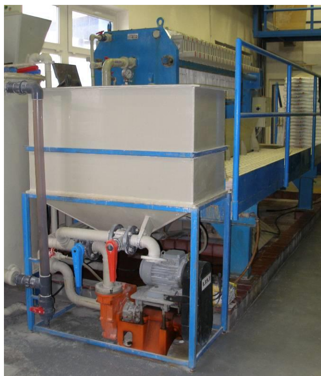
MAPE 50, Transportation of aluminium sulphate to a filter press
