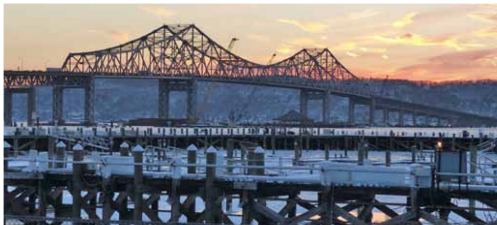
Observation de ponts (Tappan Zee Bridge USA)
