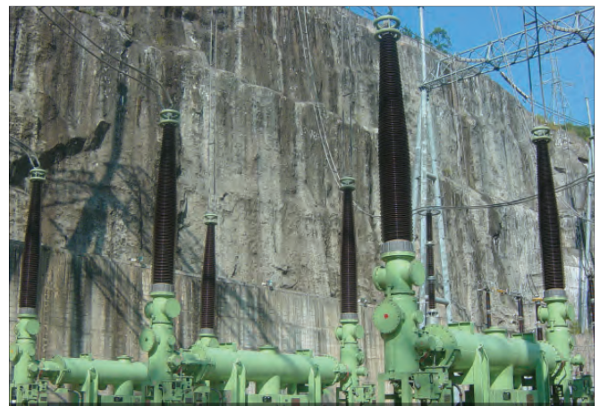
550kV Hybrid Gas Insulated Switchgear
