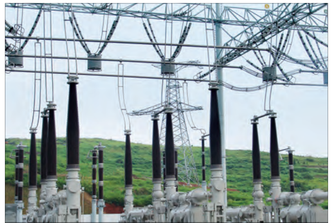
550kV Hybrid Gas Insulated Switchgear
