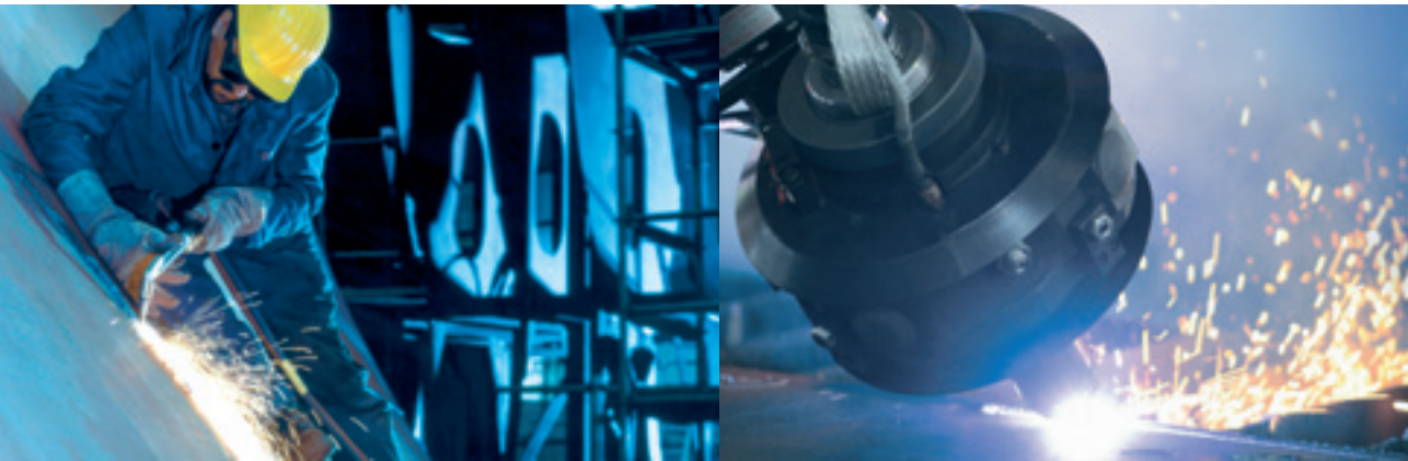
Every day tons of raw plate are cut on Messer machines and then welded by the kilometre.
